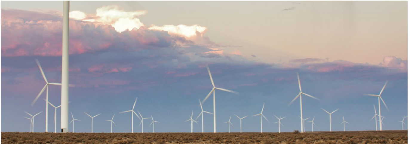
Loeriesfontein wind farm, South Africa (138MW)
