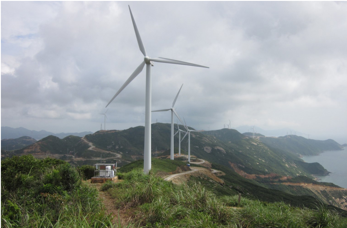
Figure 10: Example deployment within an operating wind farm in China – Photo courtesy of Longyuan Power.
